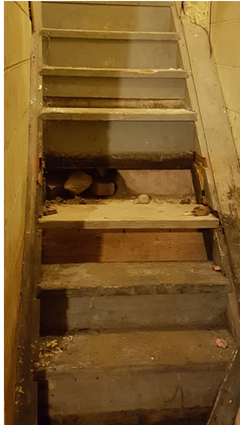
2 Basement Stairs - 4th Step Missing
