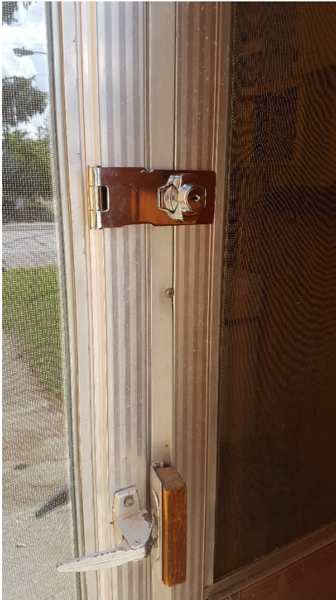
1 New Keyed Metal Latch Installed
