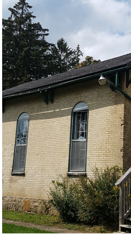
4 Eavestrough and Windows Need Repair
