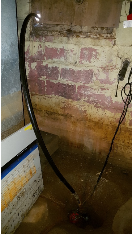
3 Sump Pump with Temporary Piping
